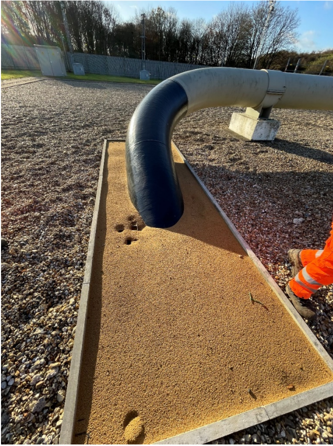
Figure 6 [REDACTED] - coating replaced on the pipework
