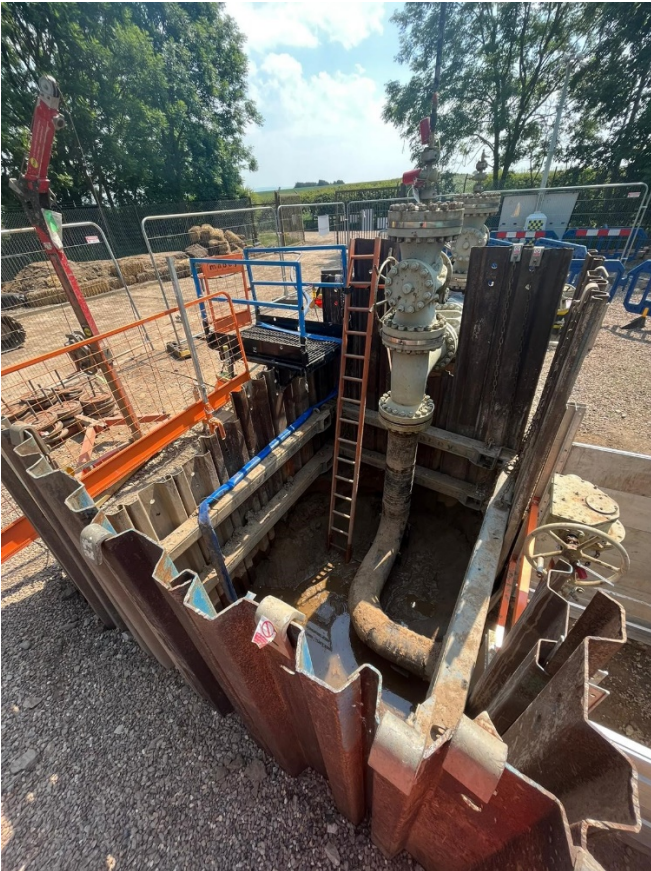
Figure 7 [REDACTED] excavation to replace damaged pipework
